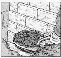
**19** Once blocks are installed, lock the first two courses in place by filling the trench in front and back with crushed stone.
